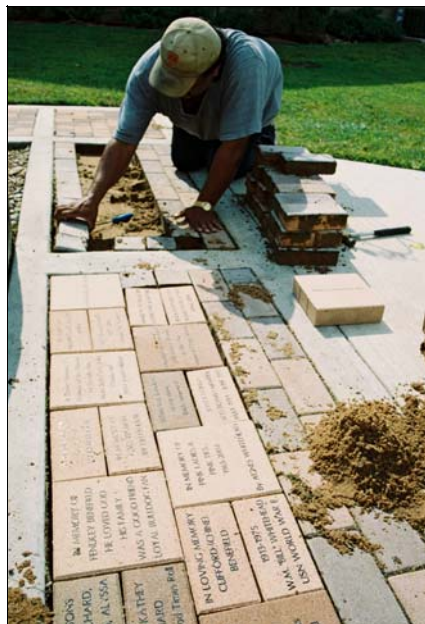
Keith Marshall installed the bricks on a hot October day.
